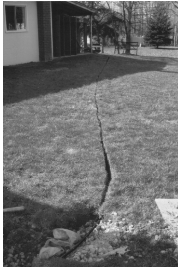
Water line placed to the pavilion.
